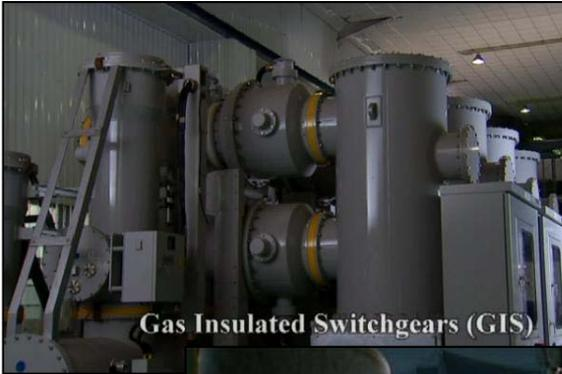
Gas Insulated Switchgears (GIS)
